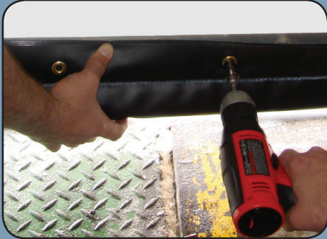
Figure 1: Edge Sealr being attached to dock door
