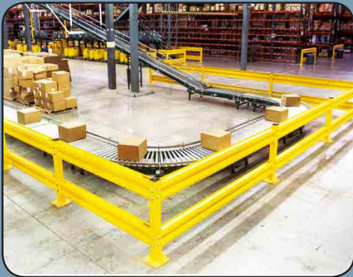
Figure 1: System of Sentry Rail installed to protect assembly process area.
