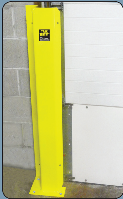
Figure 1: Trak-Sentry positioned over door tracks
